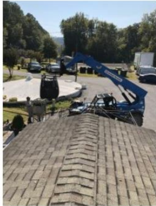
Installation in progress of new GAC filters.
