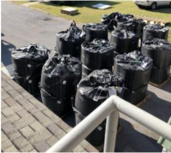
Materials for the GAC Filters at Racoon Creek.
