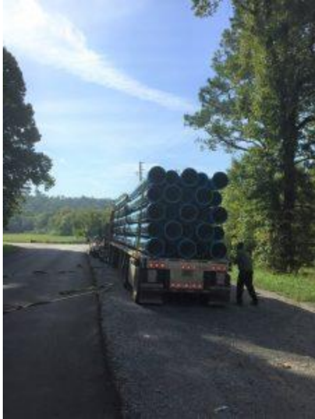
Picture above. 16" water pipe being delivered for installation.
